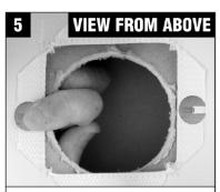
Use a hammer/screwdriver handle to open out the cover material away from the light fitting
