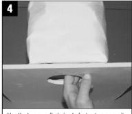
Use the two supplied pins to fasten two opposite inner flanges of the cover to the plasterboard
