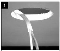
Lead the cable from the transformer through the previously-cut downlighter fitting aperture
